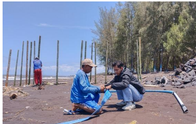
Figure 7. The on-site installation
