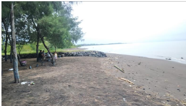
Figure 2. The existing breakwater structure
