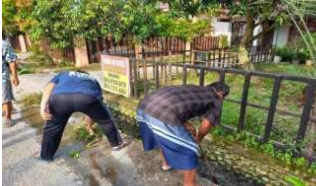
Picture 2. The cleanliness of drainage together with communities and students.
